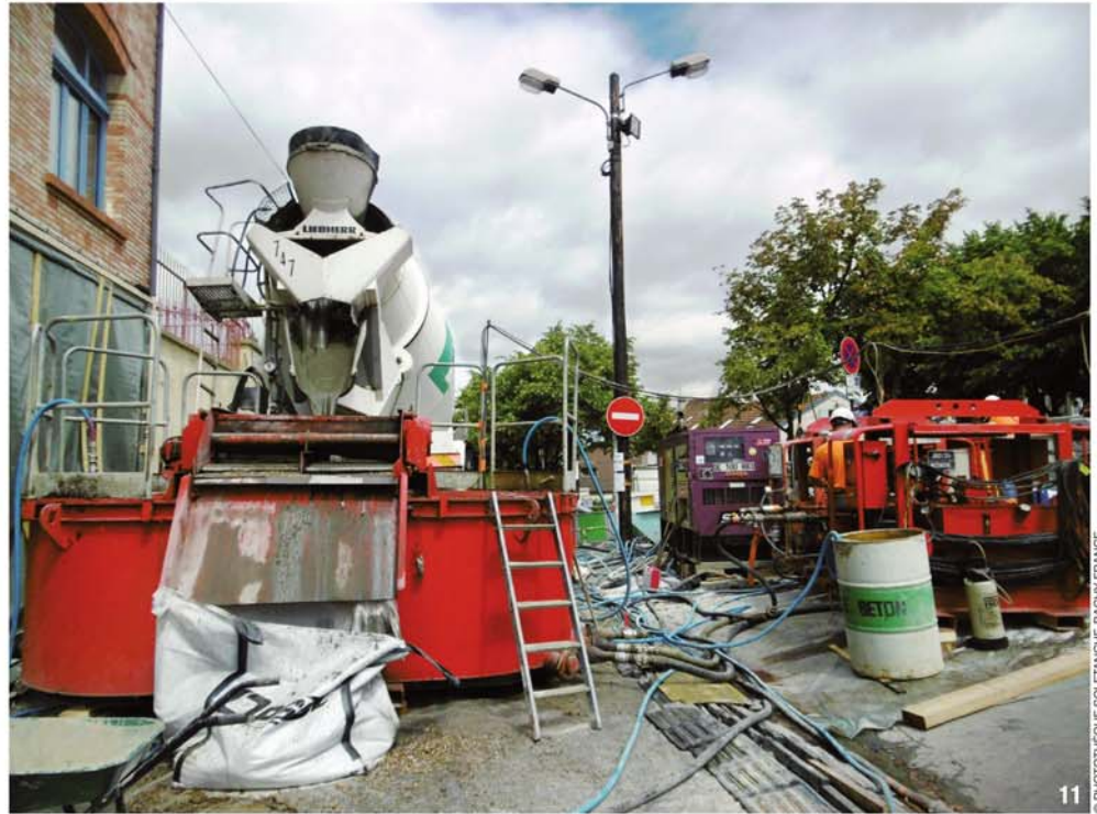
© PHOTO THÈQUE SOLETANCHE-BACHY FRANCE
