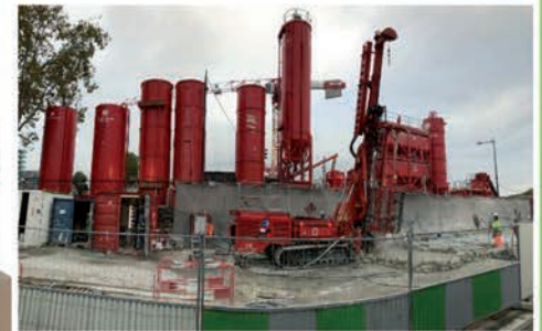
Installation chantier T3A
